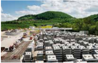
Bossler Tunnel Stuttgart / Ulm, Germany
